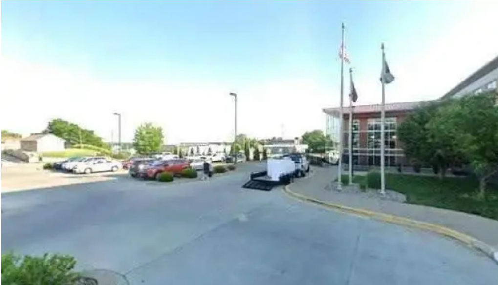
The salvation army ray joan kroc corps community center street view 360deg
